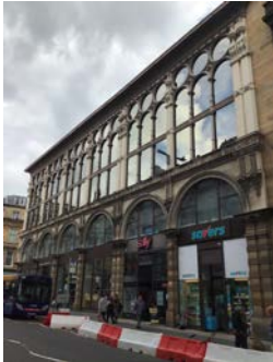
Fig. 4 The F & J Smith Warehouse (Ca'd'Oro Building), Union Street/Gordon Street 2022
