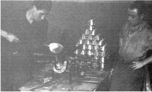
Figure 5: Hand casting aluminum parts in the Bialetti factory, c. 1930s
