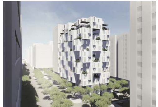
Fig. 5 The vertical kasbah in the context of downtown Abu Dhabi. The structure forms part of a continuous spatial system which includes acacia tree plantings at the foot of the structure. As the trees cast shade onto the tarmacked ground surface, air is cooled before entering the structure at the ground floor level.
