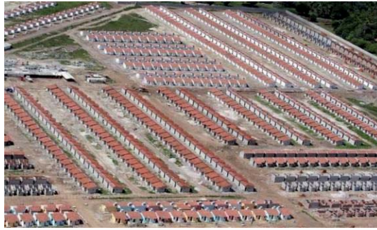
Figure 2 – An example of popular dwelling project in João Pessoa - Brazil
