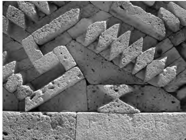
Figure 6. We can see the disposition arrange little pieces of stone block with a specific cut with angles approximate to 90°, 30°
