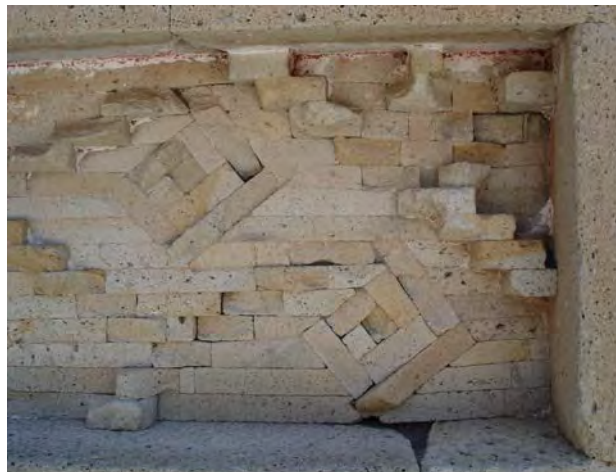
Figure 3. The accommodation of parts is arranged in bands, cut into modules.
