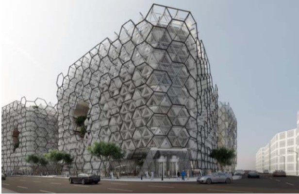
Figure 9: Mixed-use office structure [21] The project proposal was developed as a proposal to a mixed-use office structure. It was inspired by Biomimicry after an extensive field analysis. It was inspired by the hexagonal shape cell structures that dominate the façades. The façade also answers other problems. Climate control keeps pace with the city with intelligent frontage units that mechanically adapt to the sun's orbit.
