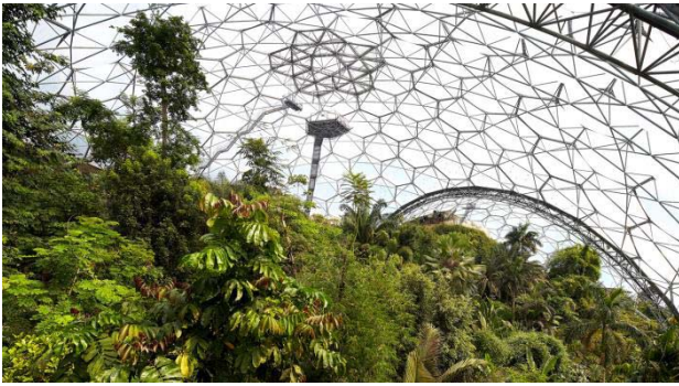
Figure 12: Eden Project roof detail [24]
